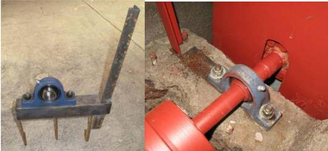
**Figure 23 – The bearing support plate before installation (left) and embedded in the concrete wall (right)**
